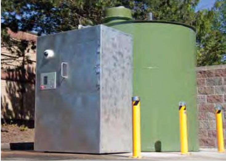
Food scraps ground up in the Harvester are pumped into the adjacent green biology tank.
