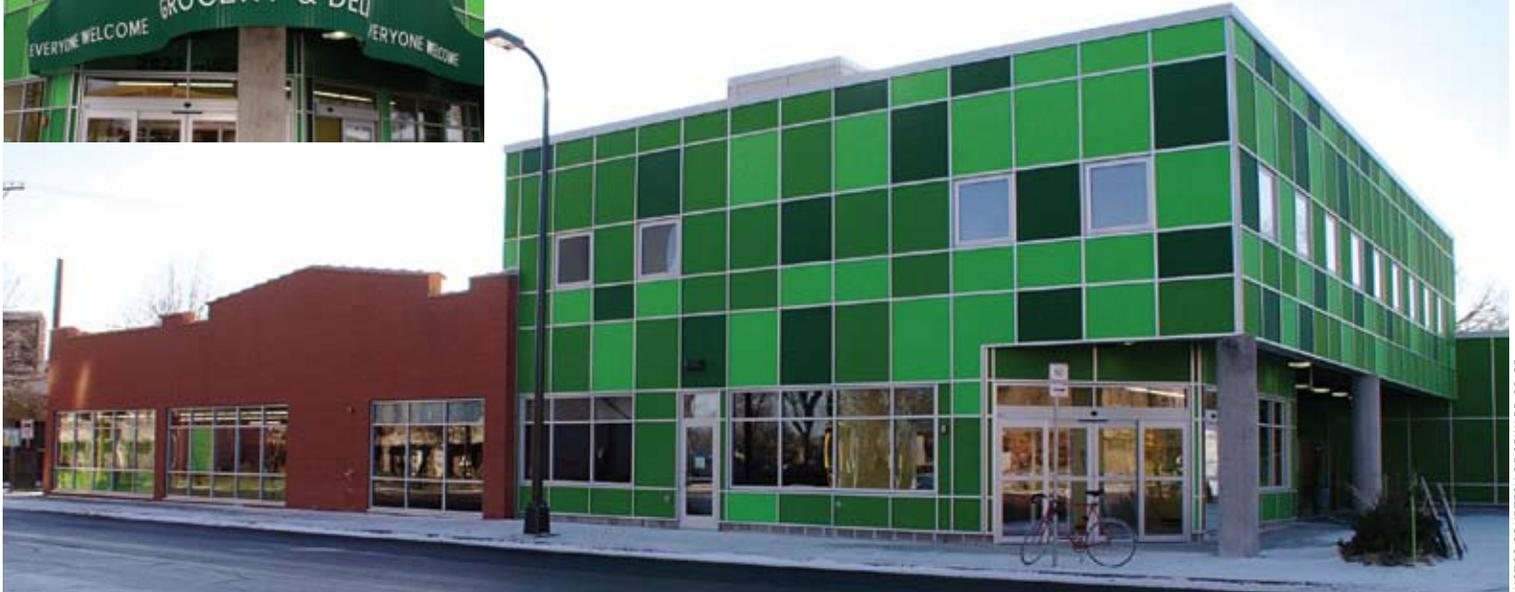
The co-op retained the shell of the former corner store (left) while constructing a two-story addition.
